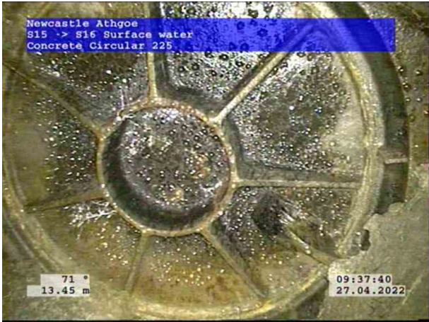
5, 00:02:06, 13.45 m Finish node, manhole, reference: S16, BURIED
