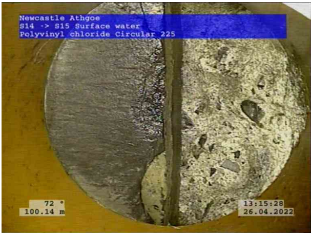
13, 00:10:48, 100.14 m Junction, closed at 2 o'clock, 150mm dia
