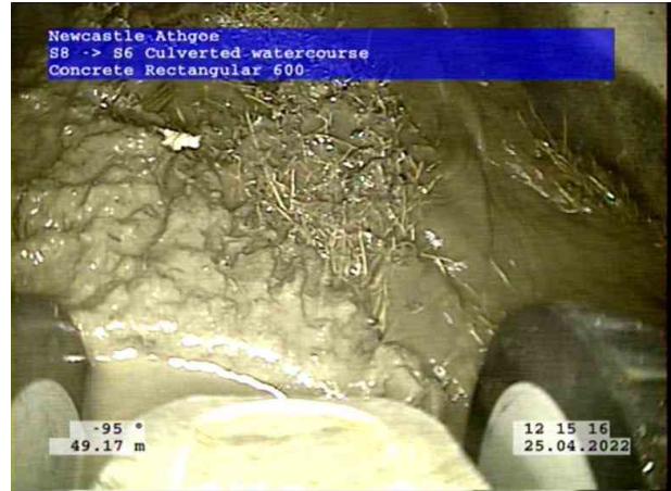
18, 00:08:51, 49.17 m Survey abandoned, UNABLE TO PASS THE ROOTS. CUTTING REQUIRED
