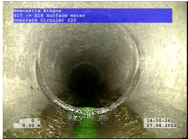
2, 00:00:06, 0.00 m General remark, SIGNS OF A DYE
