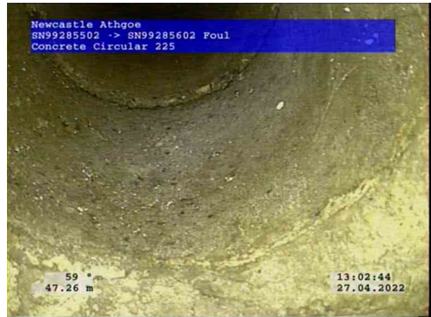
10, 00:05:32, 47.26 m Junction at 12 o'clock, 100mm dia
