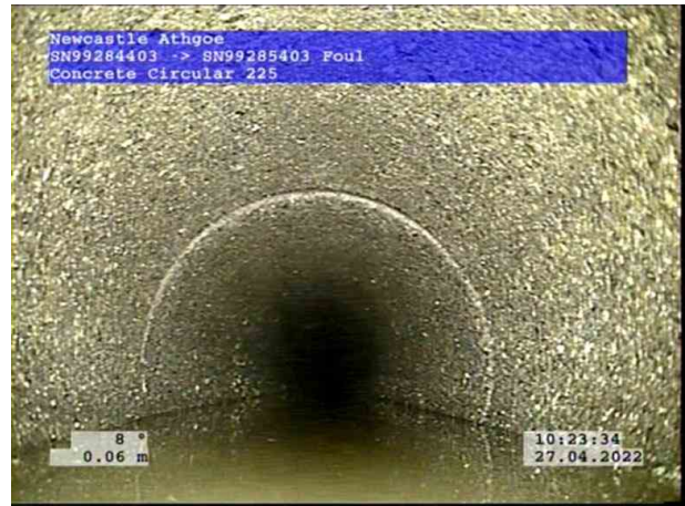
2, 00:00:07, 0.06 m Water level, 15% of the vertical dimension
