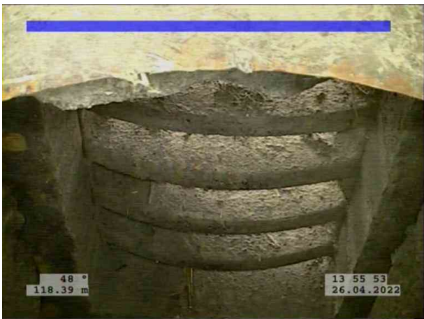
19, 00:23:51, 118.39 m Finish node, gully, reference: S15
