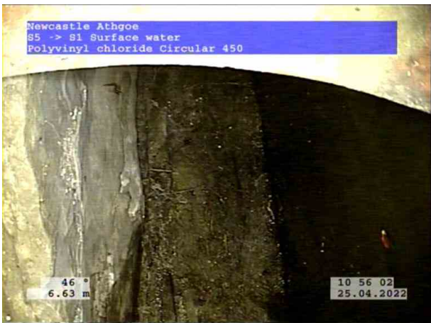
3, 00:00:53, 6.63 m Finish node, manhole, reference: S5, CULVERT
