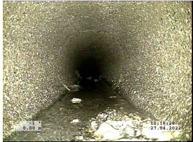
2, 00:00:07, 0.00 m Water level, 5% of the vertical dimension
