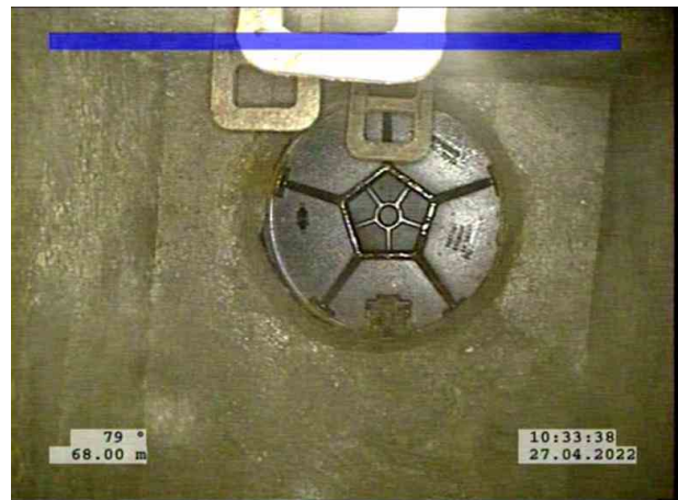
16, 00:08:12, 68.00 m Finish node, manhole, reference: SN99284403
