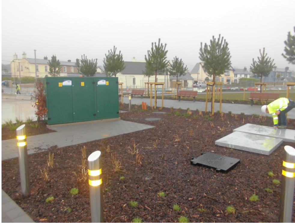
Figure 4.1 – Example foul pumping station
