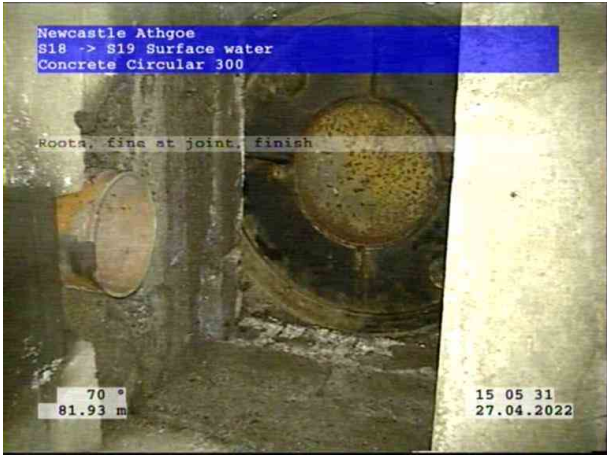
21, 00:08:15, 81.93 m Roots, fine at joint, finish
