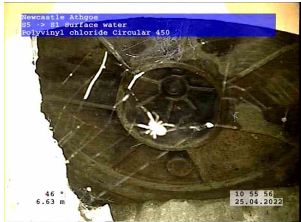
2, 00:00:53, 6.63 m Finish node, manhole, reference: S5, CULVERT
