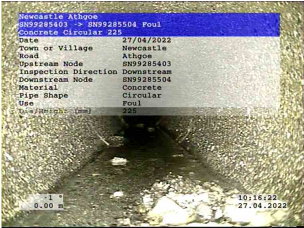
1, 00:00:00, 0.00 m Start node, manhole, reference: SN99285403
