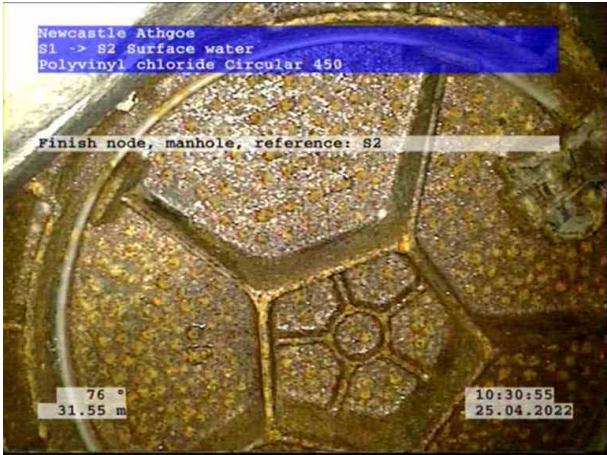
5, 00:03:56, 31.55 m Finish node, manhole, reference: S2, UNABLE TO LOCATE
