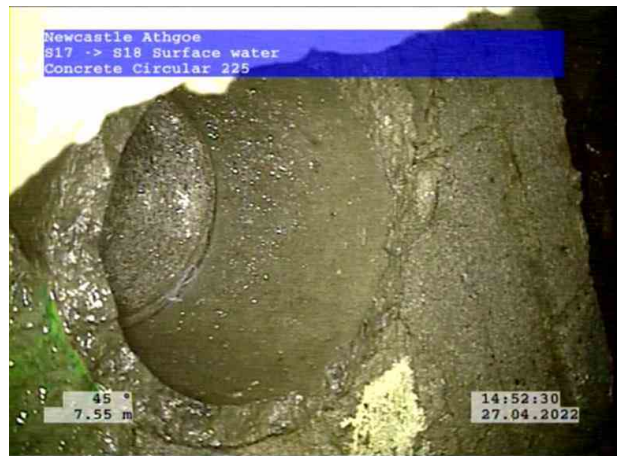
8, 00:01:18, 7.56 m Finish node, manhole, reference: S17, BURIED
