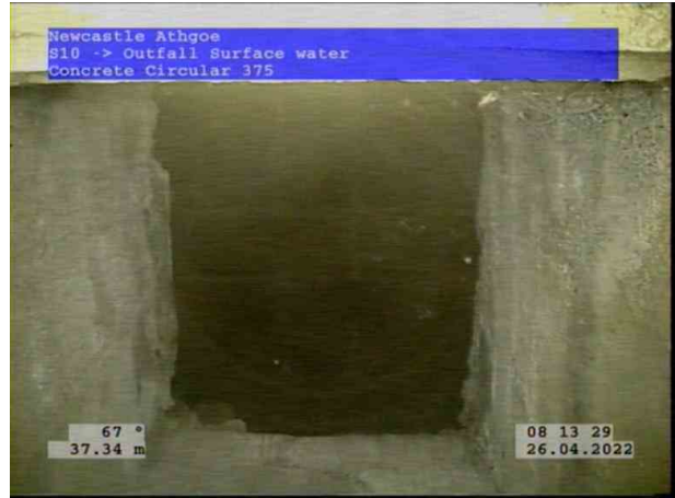
2, 00:04:08, 37.34 m Finish node, manhole, reference: S10, buried
